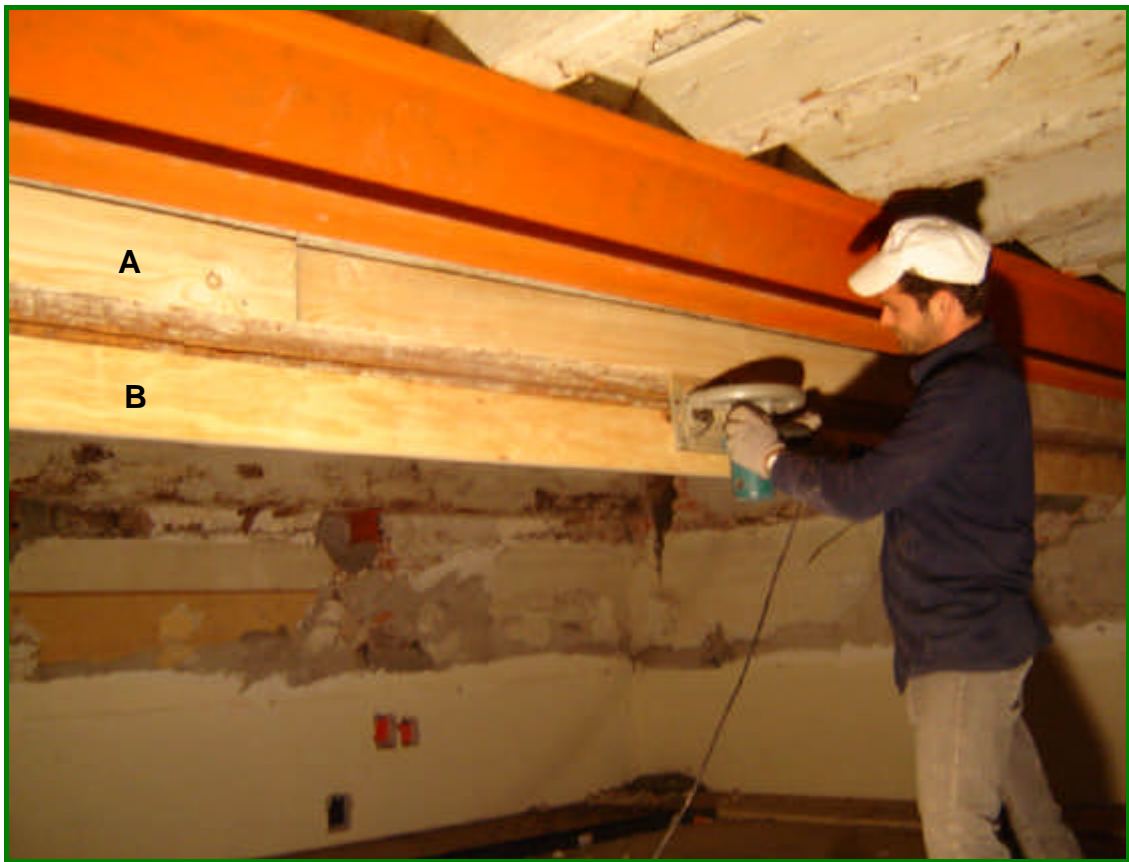
Cutting slots: an upper side guidance (A) and a lower anti-tilting support (B), made with 25 mm plywood, are fixed on the beam.
